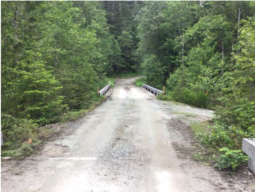
Approach from Left Bank when facing downstream
