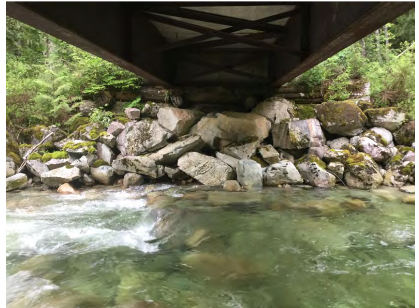
Right Bank Abutment when facing downstream
