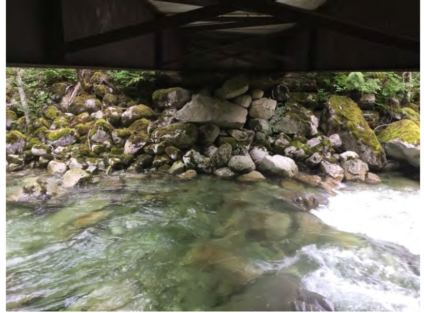
Left Bank Abutment when facing downstream
